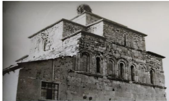
Figure 12. Unauthentic extension to narthx, 1976 (Archives of Konya Regional Dir. of Foundations).
