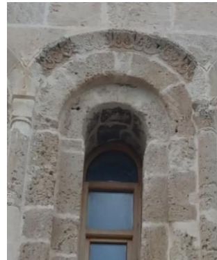
Figure 19. South Façade Arch Detail.
