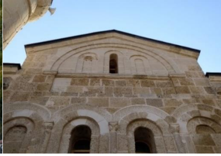
Figure 17. Detail of North Façade.
