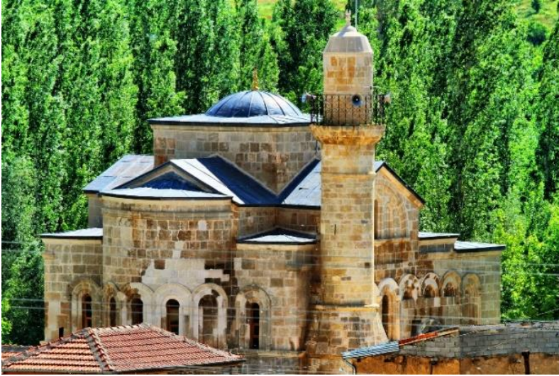
Figure 2. Fisandon Mosque General View (Anonymous).
