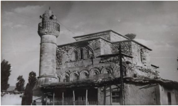
Figure 9. North Façade 1976 (Archives of Konya Regional Dir. of Foundations).
