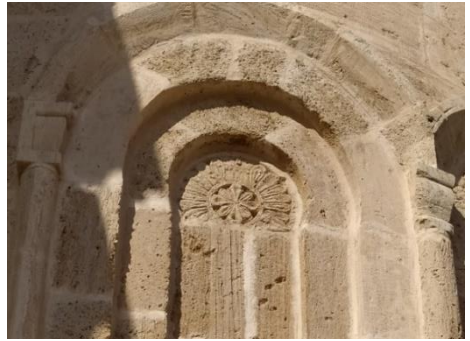
Figure 23. East Façade details after restoration.
