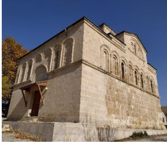
Figure 13. Narthex door and western façade.
