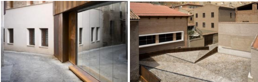
Figure 16. Street Façade (URL 23), Figure 17. Roof Surface (URL 23)
