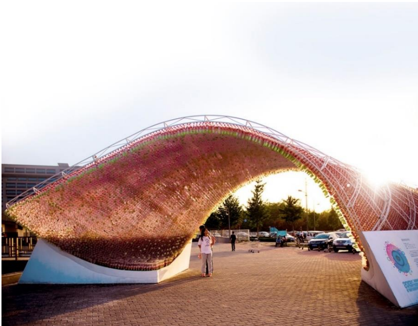
Figure 1. 'The Cola-Bow' Exterior View (Photo: Penda, URL-1)
