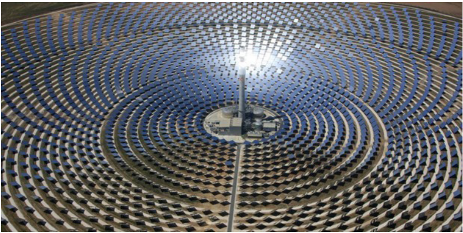
Figure 5: It Shows 5 MW Solar Power Tower in Mersin, Türkiye
