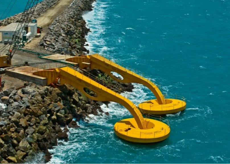
Figure 12: It Shows the Brazilian Power Plant that Produces Electricity Using Wave Action
