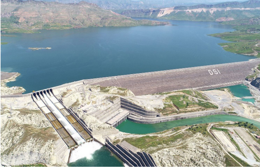
Figure 11: The Ilisu Dam and the 1.2 GW Hydroelectric Power Plant Built in Mardin-Türkiye.
