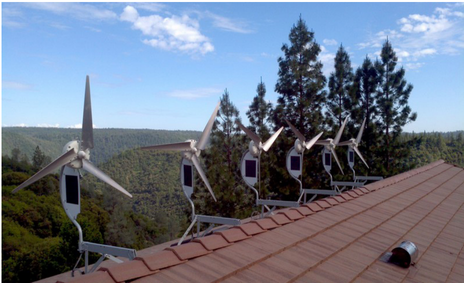
Figure 9: The Photography Shows the Wind Turbines Installed on a Home's Roof for Personal Electricity Production
