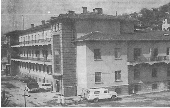
Figure 2: Izmit State Hospital (Planning - Construction period 1945-1952) ( https://kocaelidh.saglik.gov.tr/TR,115541/tarihce.html , Access Date: 09.03.2023).
