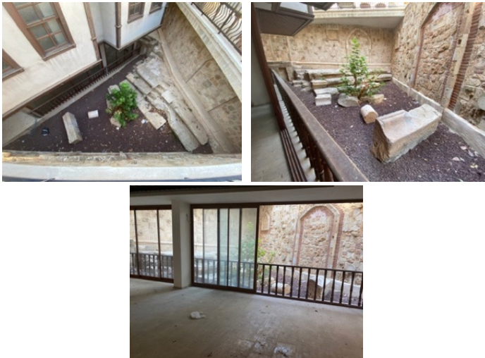
Figure 11. Photographs of the building located on 148 block 31 parcel (Original, 2021)
