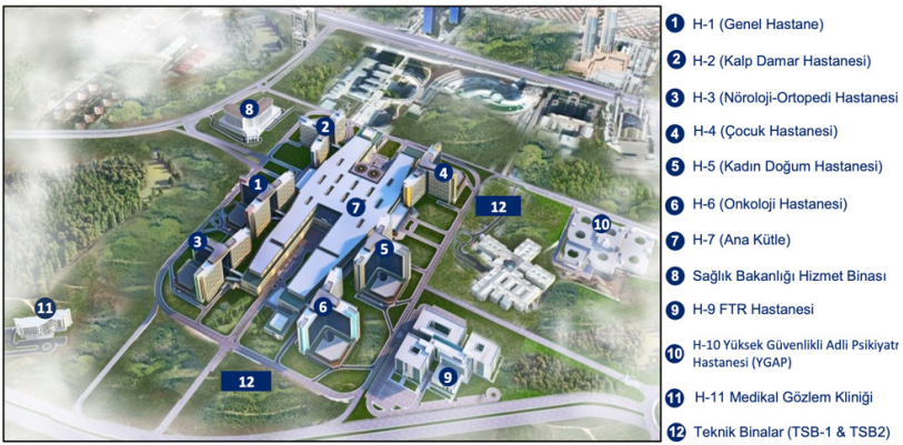
Figure 11: Ankara City Hospital campus buildings and architectural organization ( https://www.turkiyokimiyadernegi.org.tr/upload/48/Dosyalar/tmp/201959174414.pdf , Access Date: 11.03.2023).
