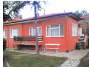
Figure 2: Sümerbank Cloth Factory Housing, (Arkitekt Journal)
