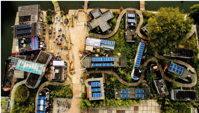
Figure 1. De Ceuvel transformation project (Deceuveel 2024)
